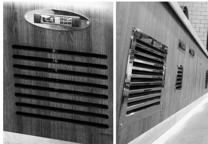
Figure 3-1. Air vent removal for cleaning – on custom counters the design of the grill will vary from the one illustrated.
